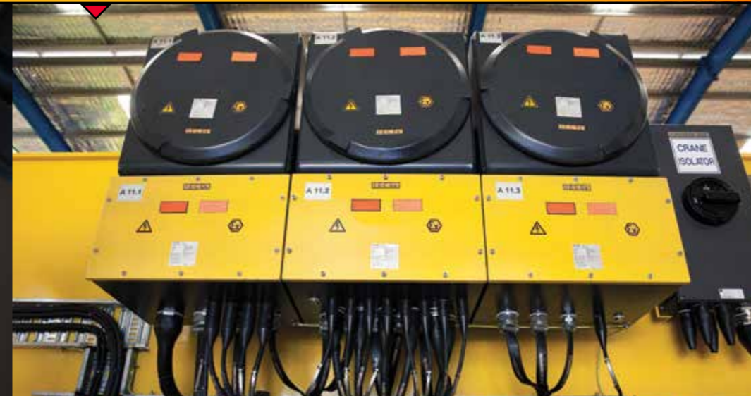
Flameproof Enclosures to increase safety
