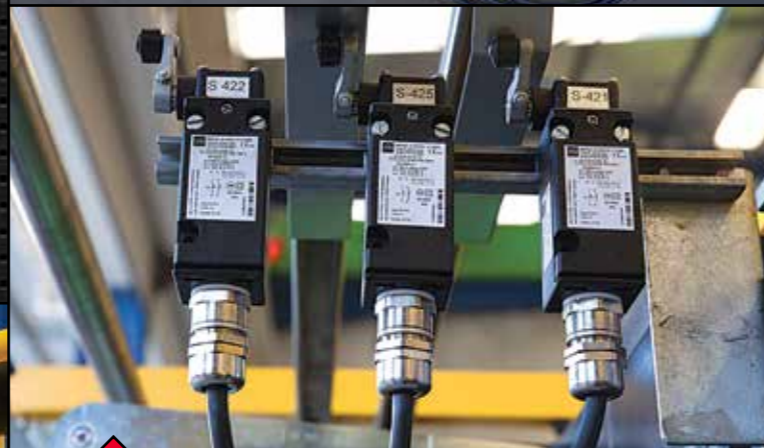
Flame-proof Limit Switches increase safety
